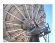
**Vertex Antenna De-Icing Control**, manual or auto mode, 120 VAC, 50 Hz Separate on/off for reflector and feed Ice detection warning and fault indicator light
